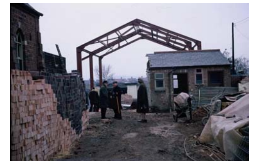
Construction in progress 1968
